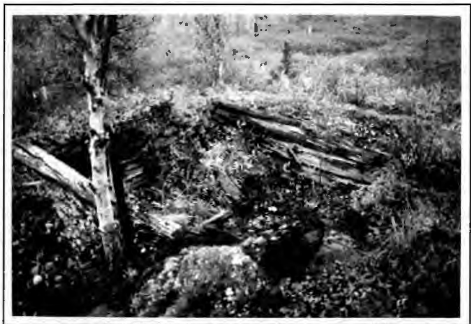
Figure 83. The entry to the Underground Cold Storage Facility, 1993. The view is looking north.
